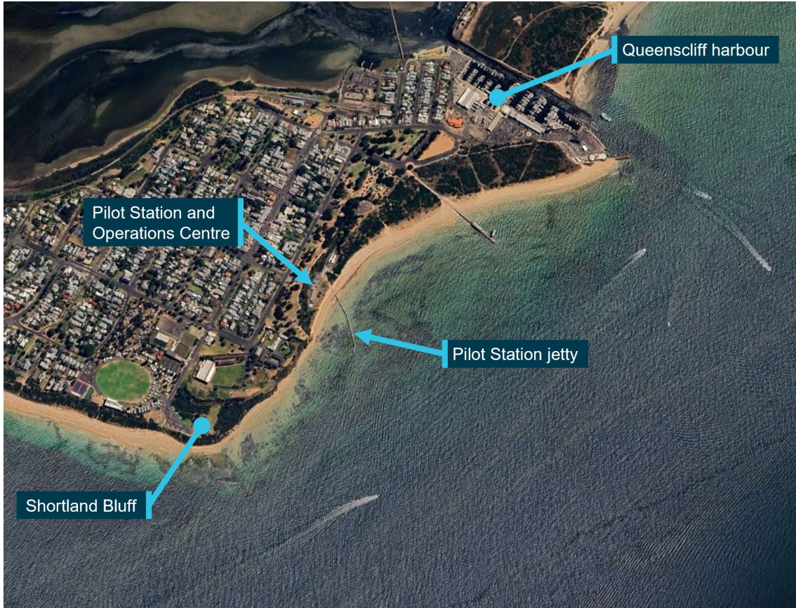
Figure 18: Location of PPSP pilot station and jetty in Queenscliff
