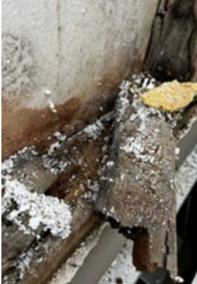
Bottom plate of timber framed balustrade.
