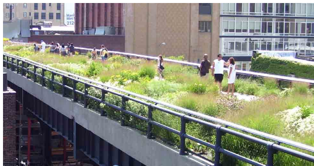
Decked park above tram tracks
