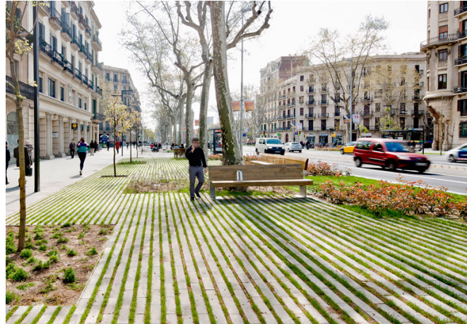
Permeable paving + underground storage
