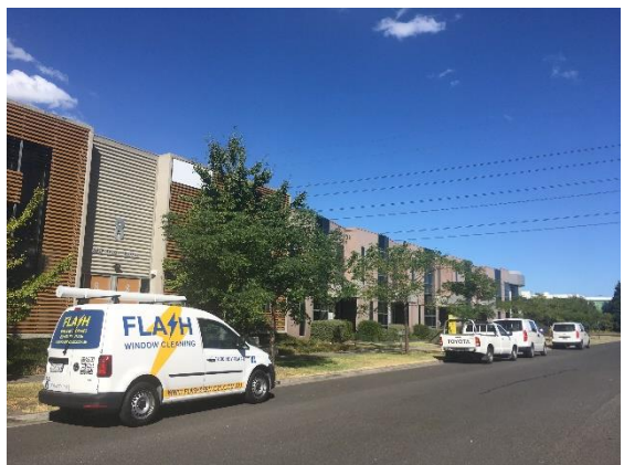
Picture 5 – 4-8 Rocklea Drive, opposite site to the east
