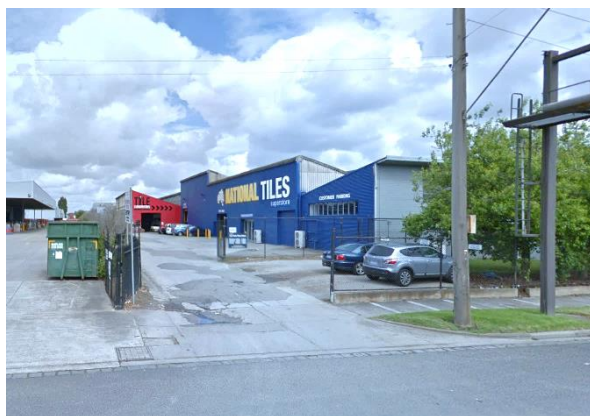
Picture 5 – 525 Graham Street, abuts the site to the south
