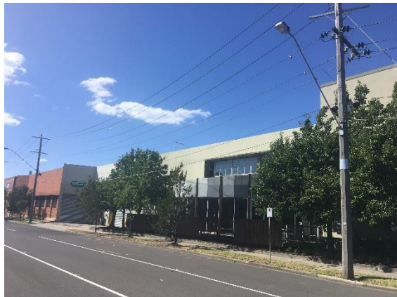
Picture 3 – 520-533 Graham Street, directly opposite the site
