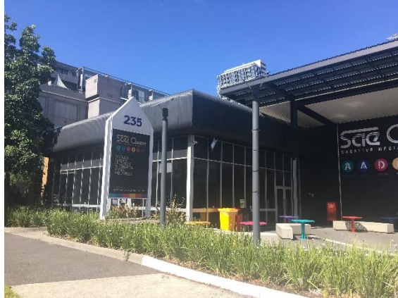
Picture 1 – 235-243 Normanby Road looking east
