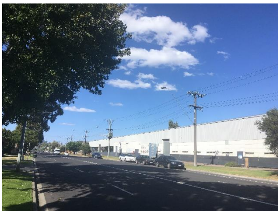
Picture 5 – 332 Plummer Street, site immediately east of subject site
