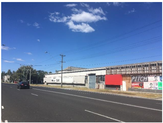
Picture 5 – 19 Salmon Street (looking east)
