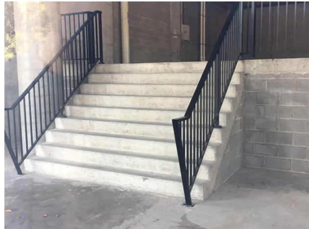
Figure 4: Gravity Tower ground floor tenancy (from Gladstone Street) with internal stair to approximately 1.7-1.8m in height.
