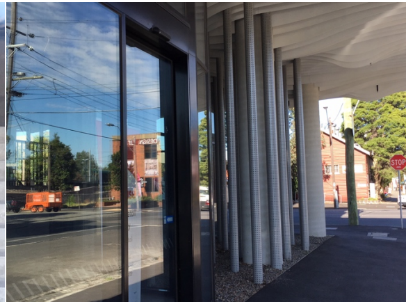
Figure 6: Gravity Tower ground floor frontage to Gladstone Street, with wind amelioration devices (vertical perforated pipes).
