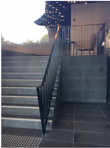
Figure 3: Gravity Tower main entrance, taken from outside the glass doors.
