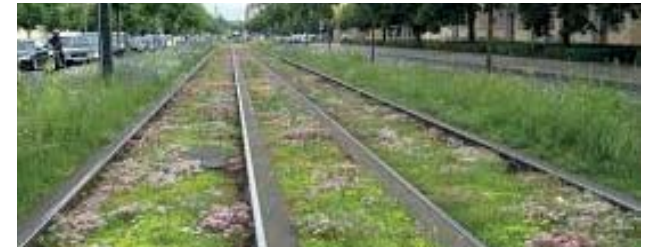
Green tram tracks add to the overall green infrastructure.
