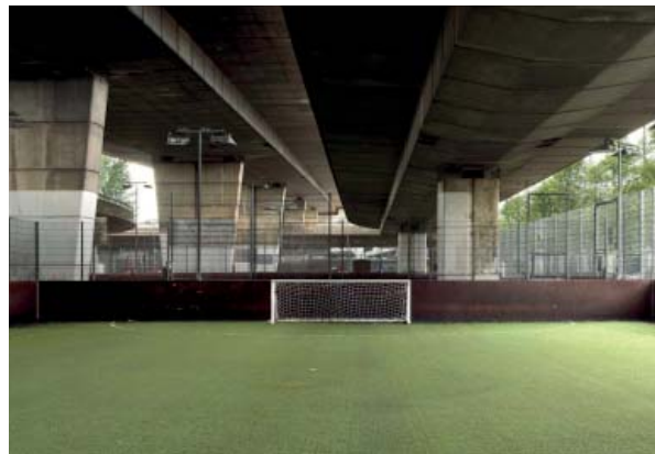
Active uses underneath bridge structures
