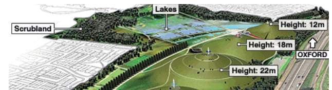
Northala Fields- new park created from construction waste.
