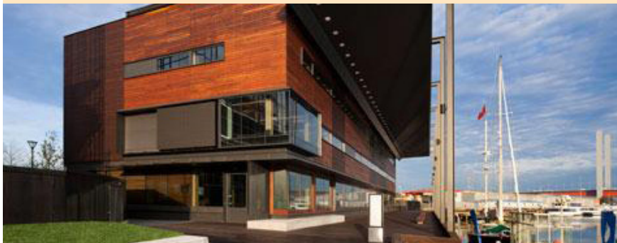
Figure 4: Library at the Dock, Community facility, Docklands, Victoria
