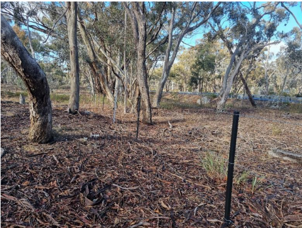
Photo 6 Fence condition along Old Glenorchy Road.
