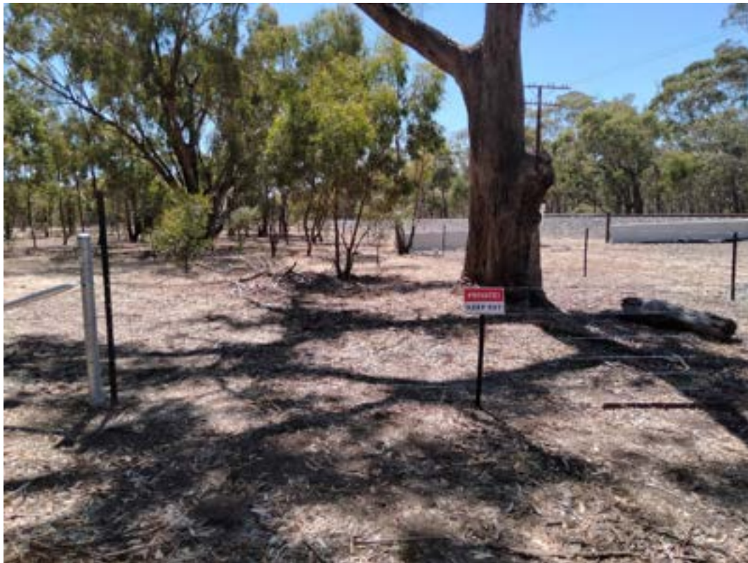
Fence Installation – South East Corner Mallee Gate (Feb 2022)
