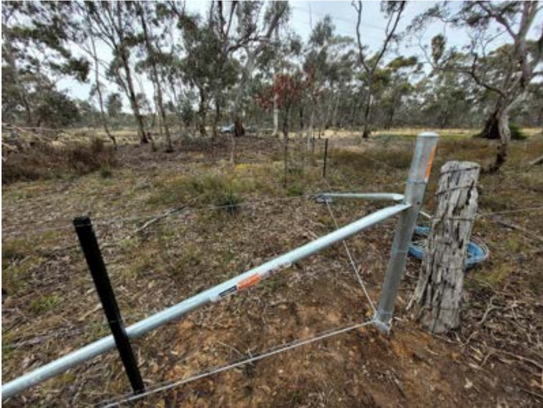
Fence Installation – South-west Corner – November 2021
