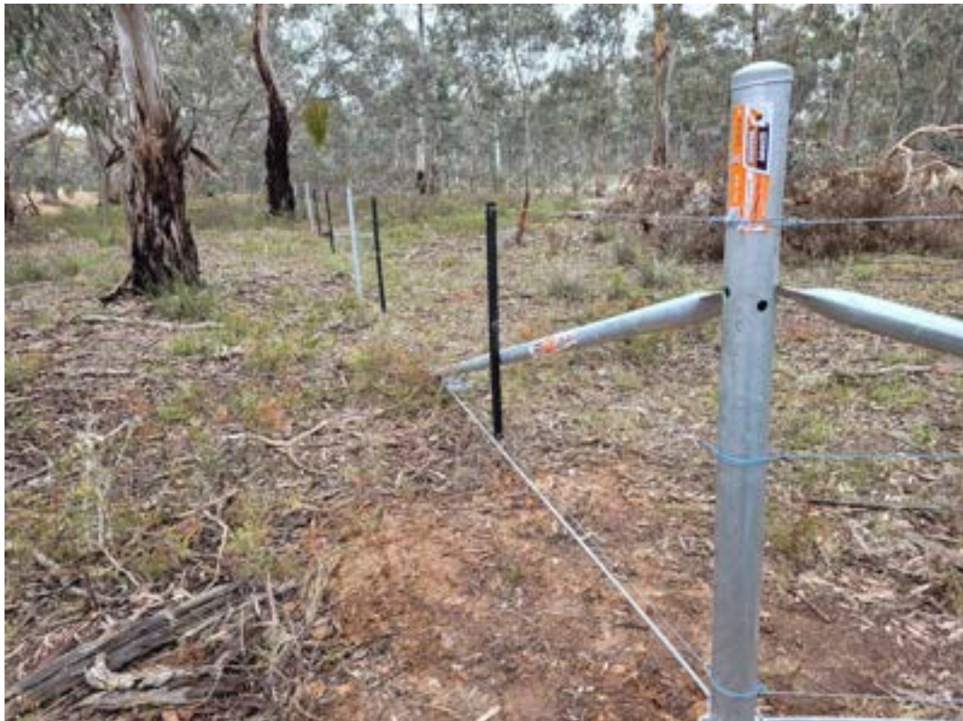
Fence Installation – North-west Corner - November 2021
