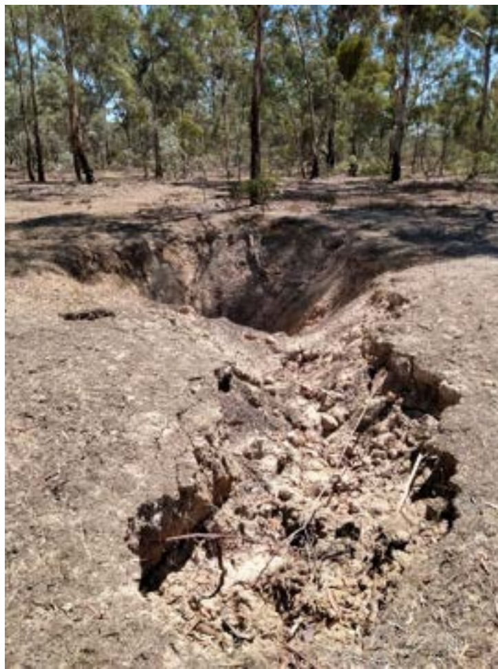
Collapsing mineshaft – February 2022 HZ 1A/1D – East of easement – February 2022
