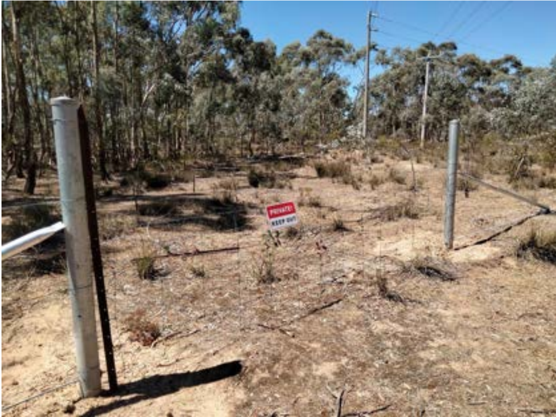
Fence Installation – South West Mallee Gate - February 2022
