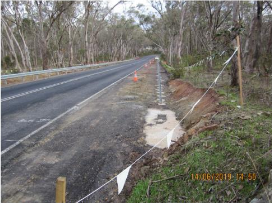
Plate 17. Pyrenees Hwy (Sec 2) Ch 12.560 – 12.445 km RHS, Limits of Works, 14 th June 2019.
