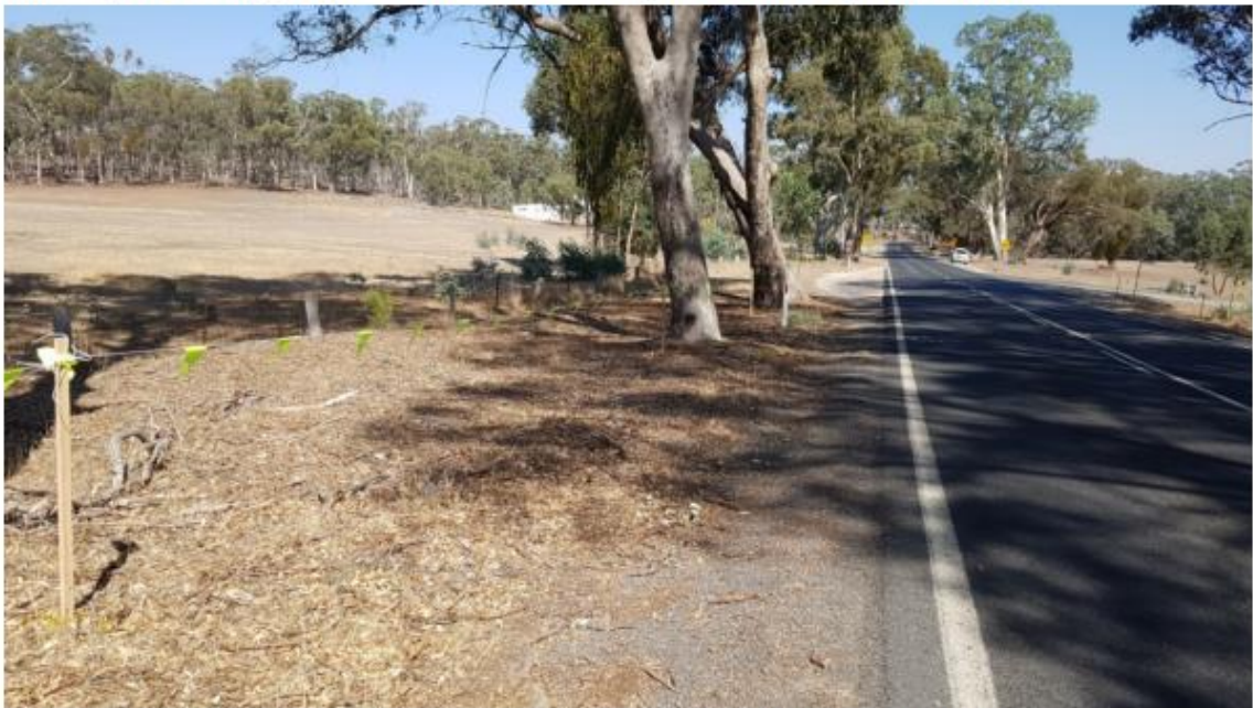
Plate 6. Pyrenees Hwy (Sec 2) Ch 14.720 – 14.880km HHS, Limits of Works, 7 th March 2019.
