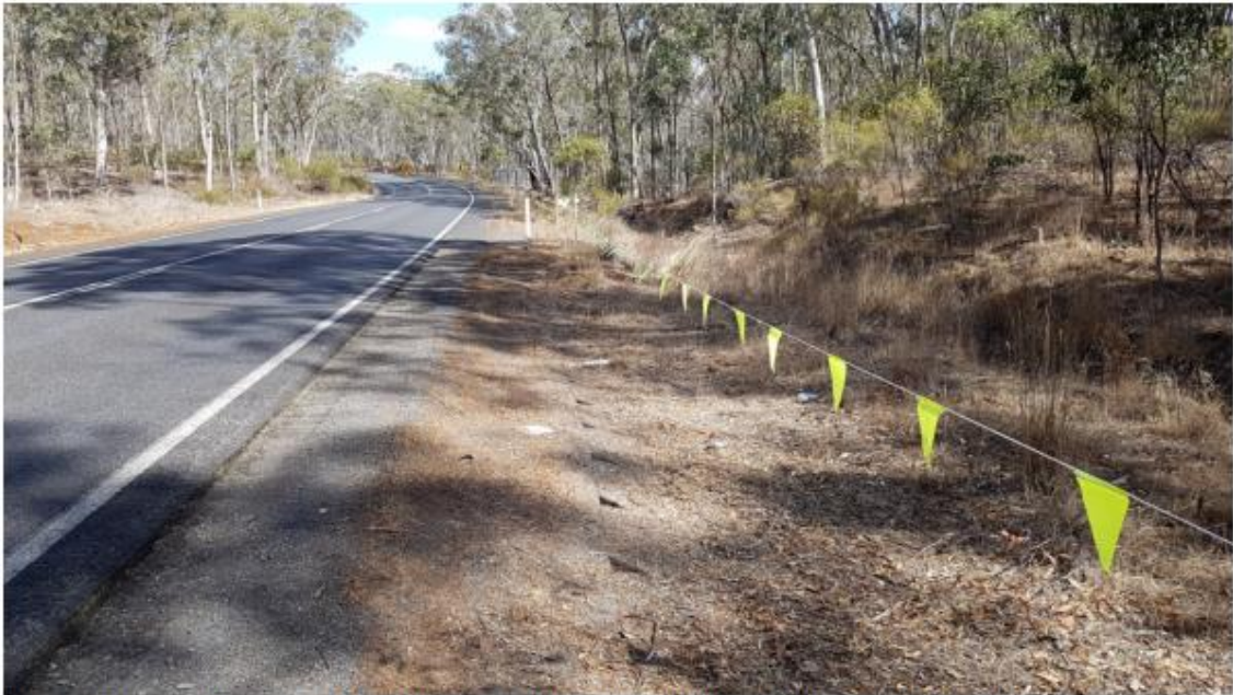
Plate 1. Pyrenees Hwy (Sec 2) Ch 11.125 – 11.390 km RHS, Limits of Works, 7th March 2019.
