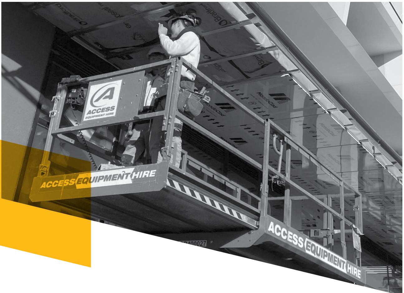
Image: A building with works underway in CSV's Cladding Rectification Program.
