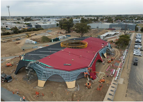
The Munarra Centre during construction.
