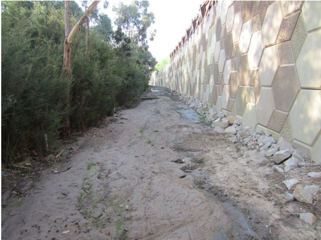
Plate 1 – Retaining walls in Pines FFR
