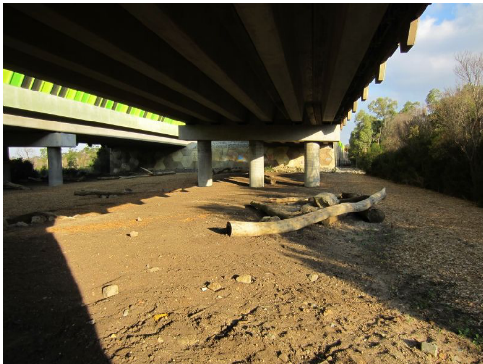
Plate 2 – Major fauna underpass (June 2012)
