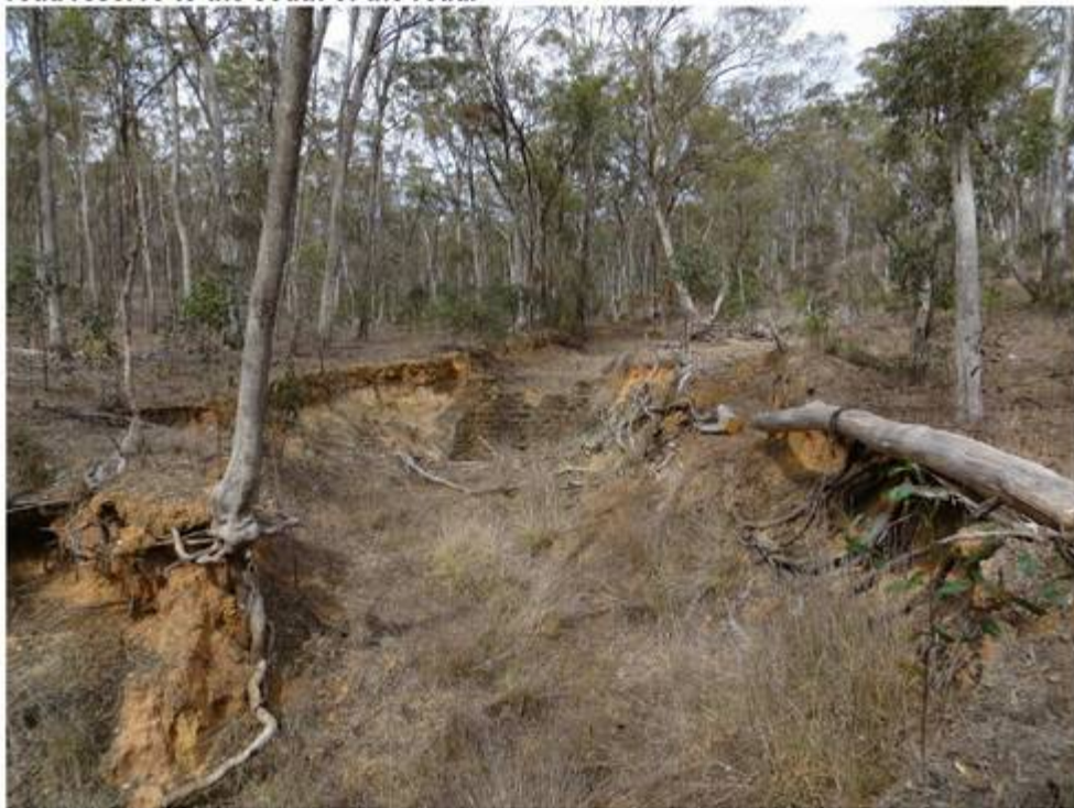
Water race feature HF001, looking west along channel towards stone and mortar water control feature (HF002)
