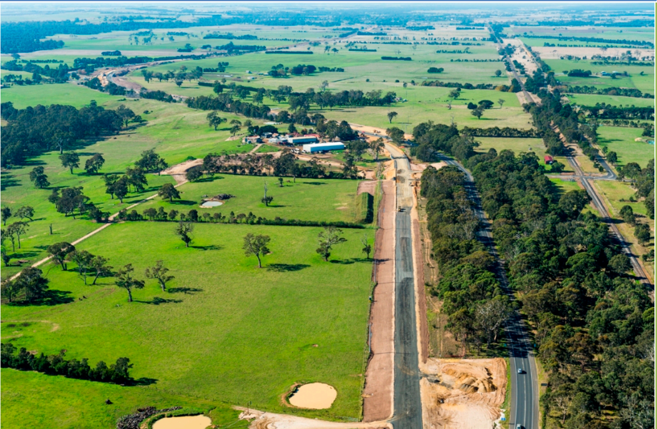
Figure 1: Aerial photograph of construction works at Flynn
