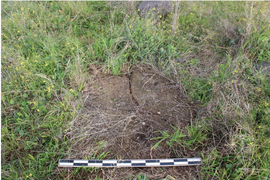
Photograph 6: In situ section of concrete floor at H7822-0160 (Drover's Hut) (K. Flemming 24.6.2013)
