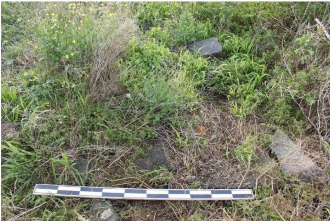
Foundations of hut - detail
