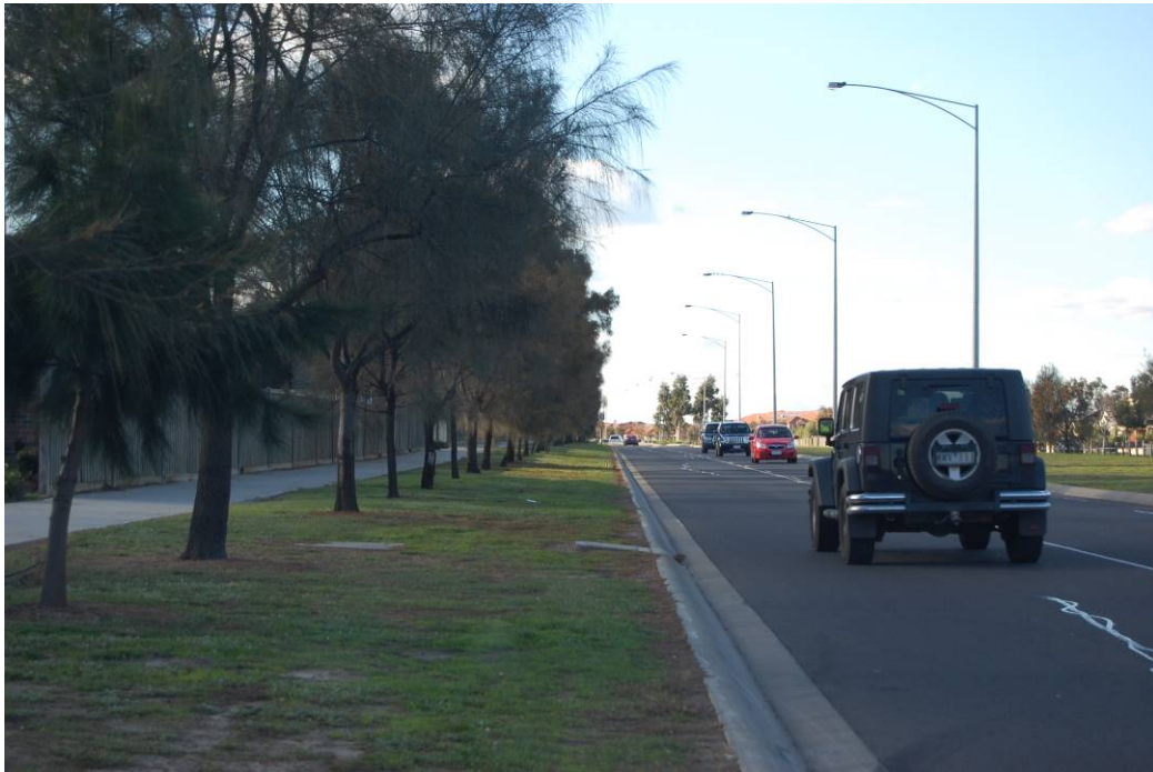
Photo 29 Street trees along Calder Park Drive that will need to be removed and cannot be replaced under the current clear zone requirements.
