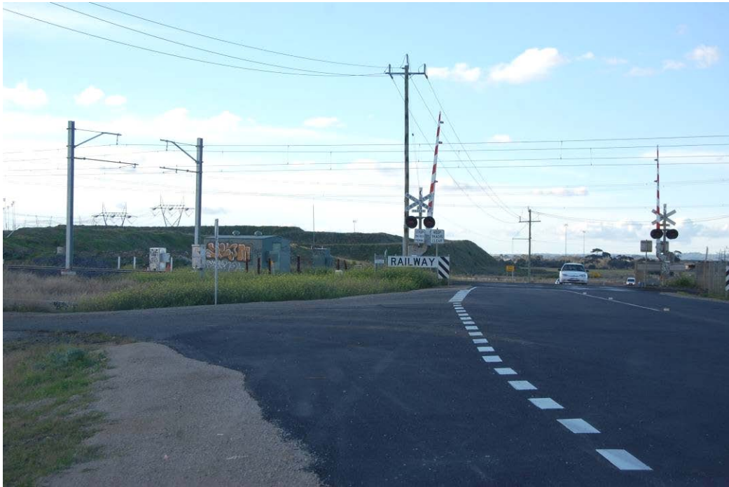
Photo 27 The location of the Melbourne-Bendigo Railway line overpass.
