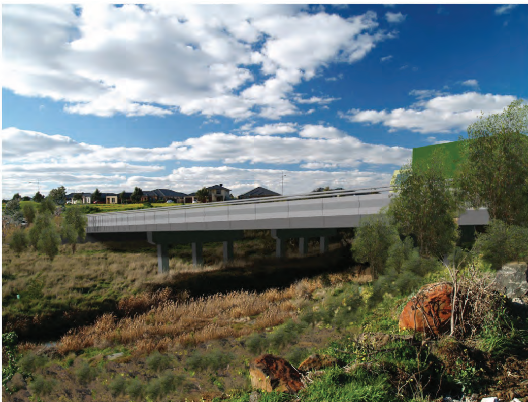
Figure 11-12 Kororoit Creek valley, looking north east: existing (top) and future mitigated (bottom) views
