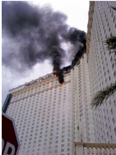
Figure 48 – Monte Carlo Casino Façade Fire (2008)
