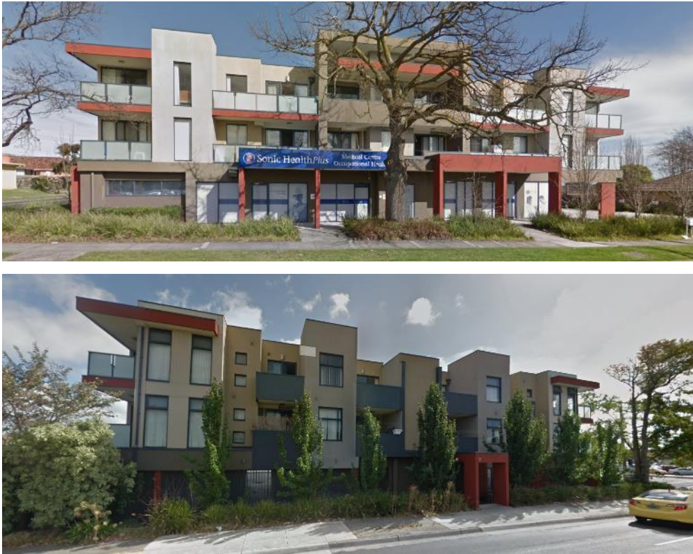
Figure 30. Street elevations of 161 Princes Hwy Dandenong (google street view)
