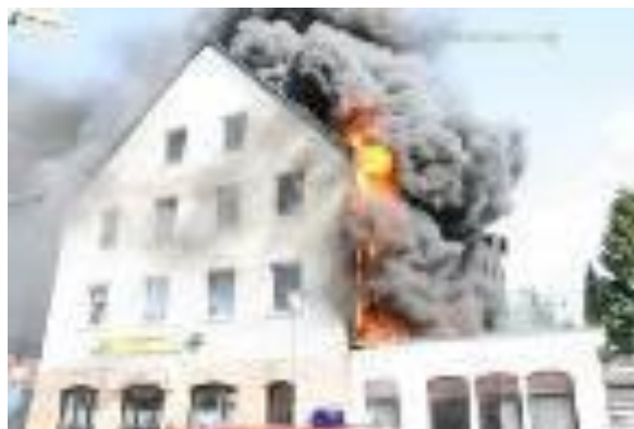
Figure 39. Aachen EIFS fire 22/05/2009 [75]
