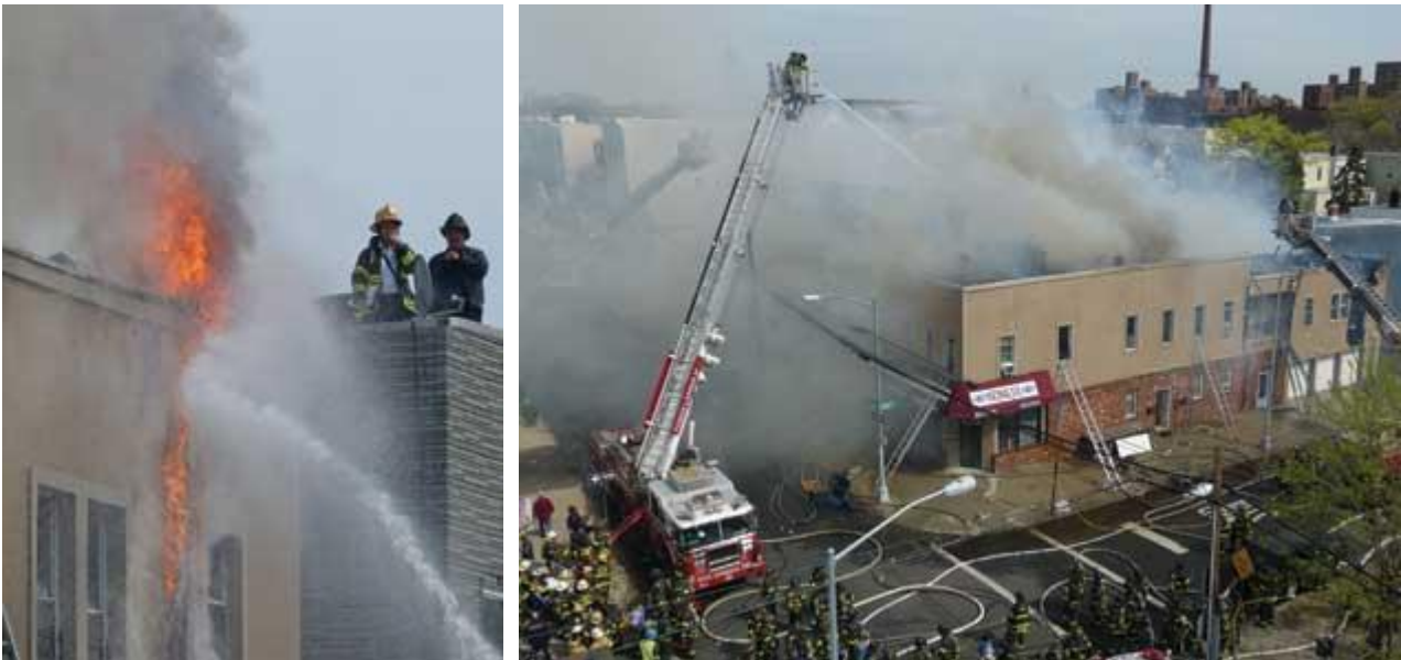
Figure 43 -Flames burn vigorously above the roof line of the EIFS-clad structure (left), View of opposite side of building (away from area of fire spread) [78]
