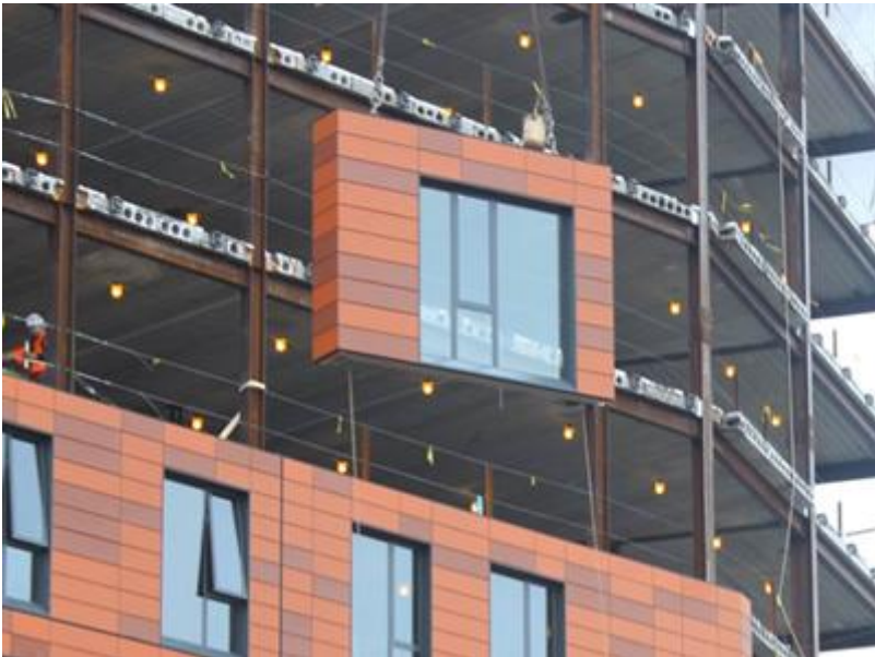
Figure 9. Unitised façade panels
