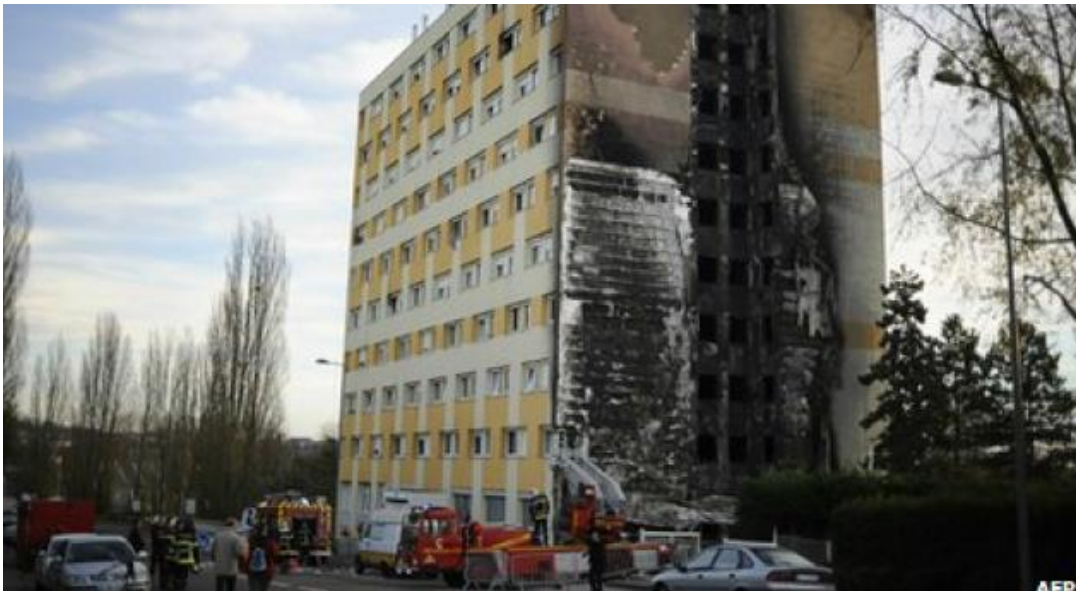
Figure 45 – Dijon France Immigrant hostel post fire damage [80]
