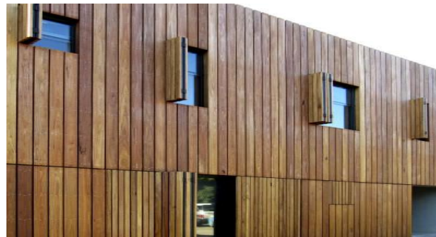
Figure 5. Typical CLT Panels (left), Forte 10 storey residential CLT building in Melbourne (right), Typical hard wood cladding (bottom).
