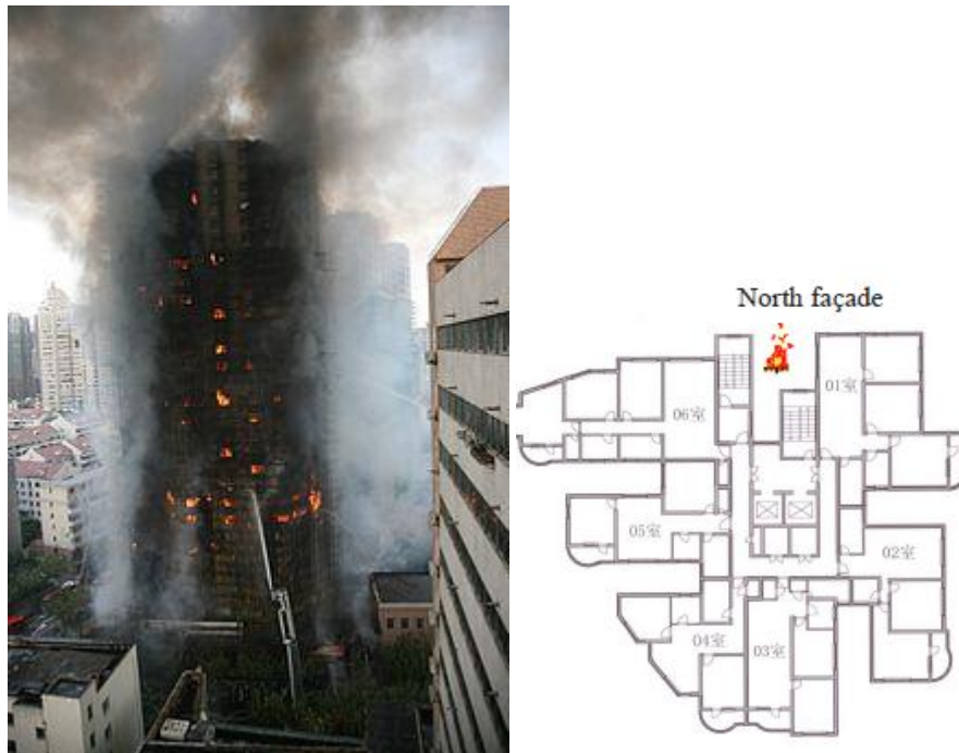
Figure 44 –Plan view of the building showing the outline of the external face of the building and location of fire. [79]
