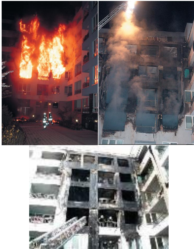
Figure 41 – The stage of the fire upon the arrival of the fire brigade (LHS) and Post fire damage (RHS and bottom) [77]
