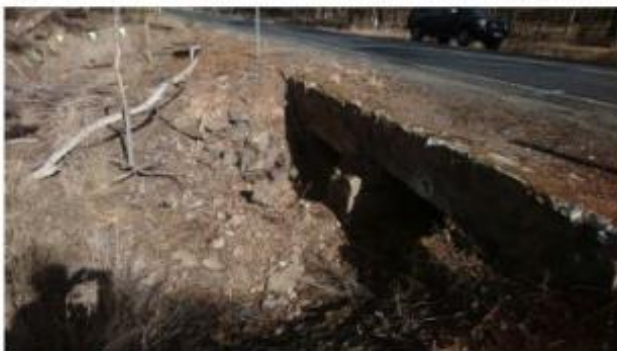
Photo 4: Pyrenees Highway, showing culvert and rocks; potential for fauna habitat (CH 11.14)
