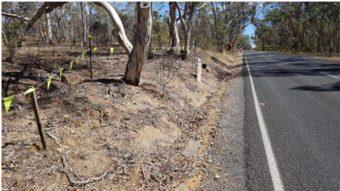
Plate 2. Pyrenees Hwy (Sec 2) Ch 12.980 – 13.325km LHS, Limits of Works, 7 th March 2019.
