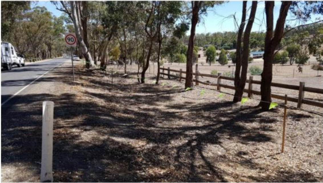
Plate 5. Pyrenees Hwy (Sec 2) Ch 14.000 – 14.070km RHS, Limits of Works, 7 th March 2019.
