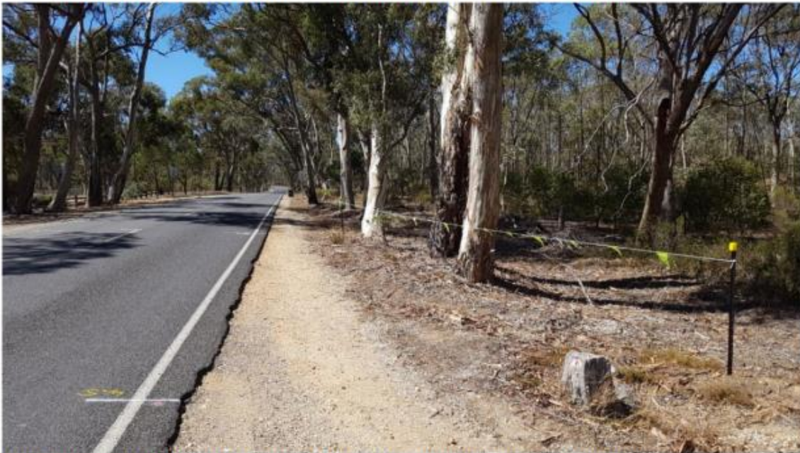
Plate 4. Pyrenees Hwy (Sec 2) Ch 13.705 – 14.065km LHS, Limits of Works, 7 th March 2019.
