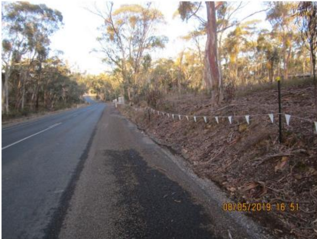
Plate 11. Pyrenees Hwy (Sec 2) Ch 13.100 – 13.325 km LHS, Limits of Works, 8 th May 2019.
