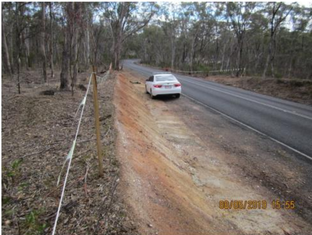
Plate 10. Pyrenees Hwy (Sec 2) Ch 12.405 – 12.570 km LHS, Limits of Works, 8 th May 2019.
