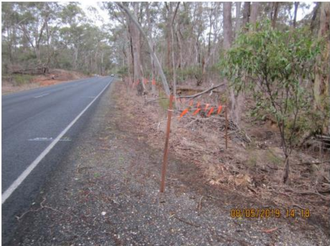
Plate 8. Pyrenees Hwy (Sec 2) Ch 10.195 – 11.047 km LHS, Limits of Works, 8 th May 2019.
