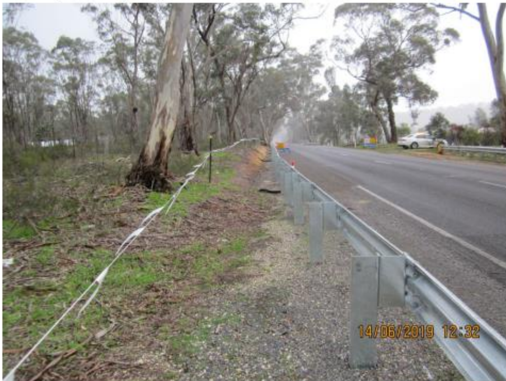
Plate 12. Pyrenees Hwy (Sec 2) Ch 13.705 – 14.065 km LHS, Limits of Works, 14 th June 2019.
