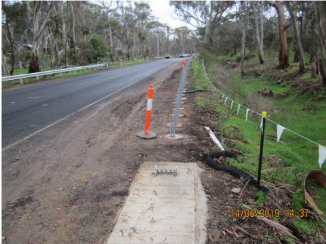
Plate 15. Pyrenees Hwy (Sec 2) Ch 13.120 – 12.995 km RHS, Limits of Works, 14 th June 2019.
