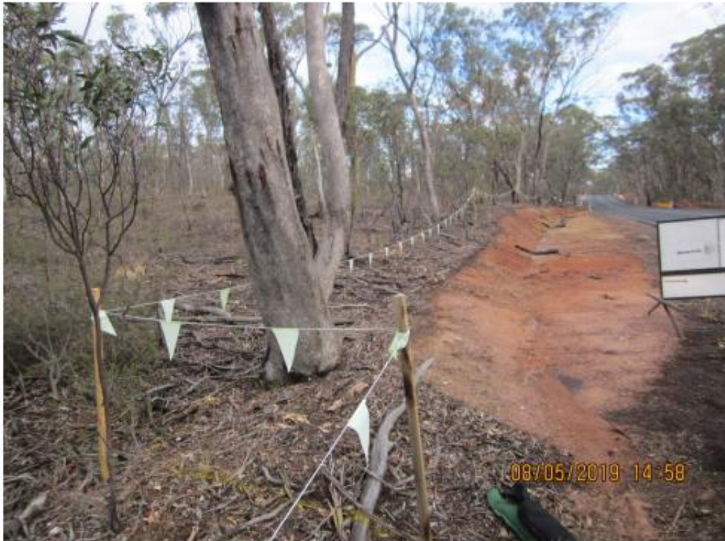
Plate 9. Pyrenees Hwy (Sec 2) Ch 11.615 – 11.880 km LHS, Limits of Works, 8 th May 2019.
