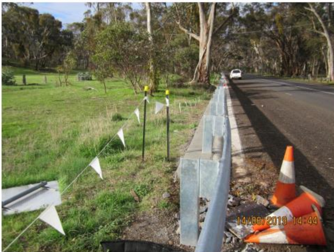
Plate 16. Pyrenees Hwy (Sec 2) Ch 12.800 – 12.575 km RHS, Limits of Works, 14 th June 2019.
