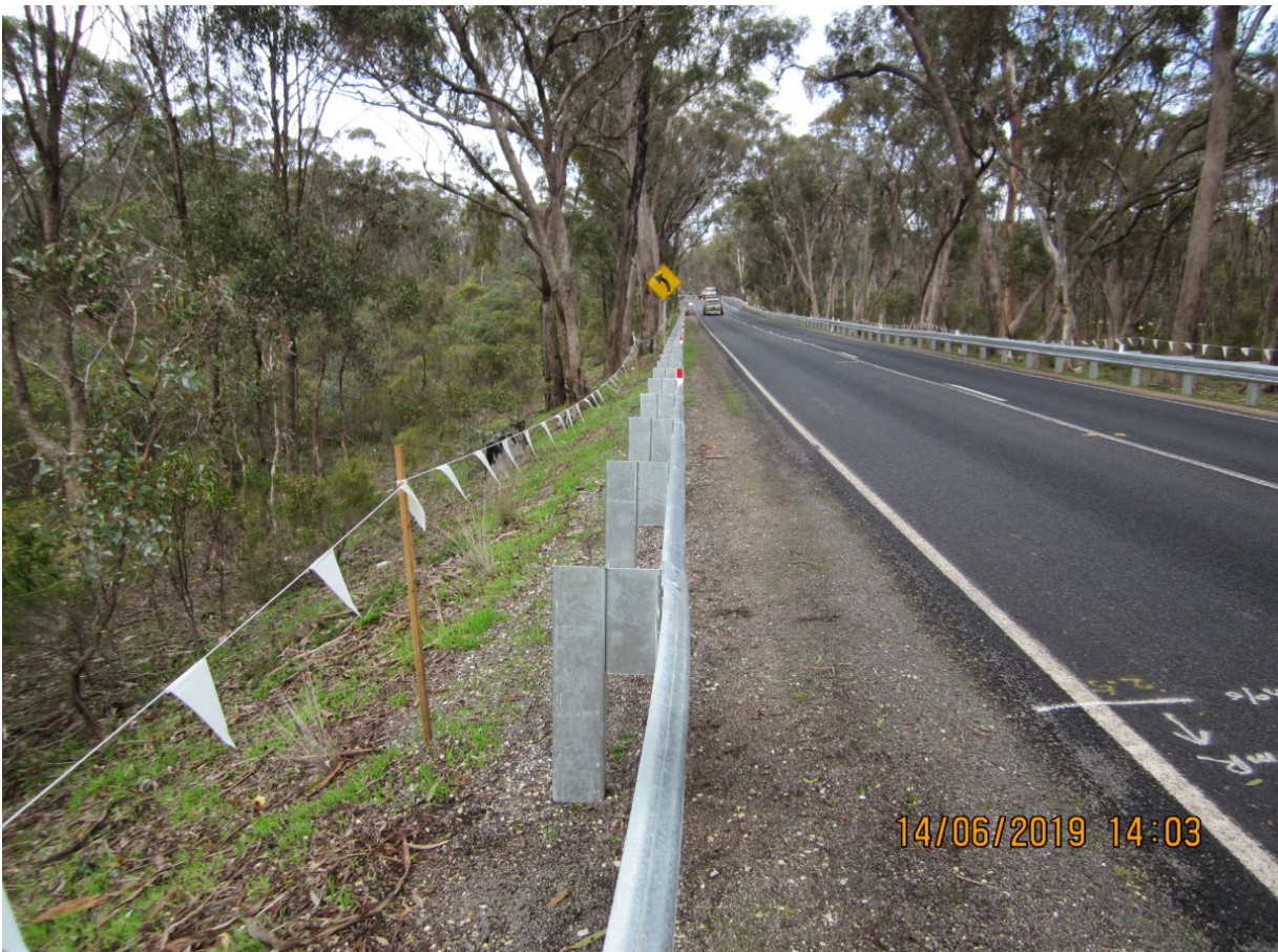
Plate 14. Pyrenees Hwy (Sec 2) Ch 13.925 – 13.700 km RHS, Limits of Works, 14 th June 2019.
