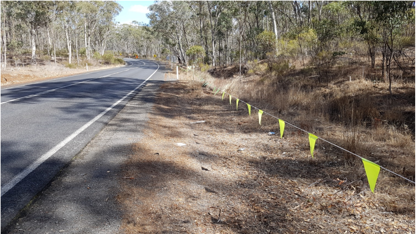
Plate 1. Pyrenees Hwy (Sec 2) Ch 11.125 – 11.390 km RHS, Limits of Works, 7th March 2019.
