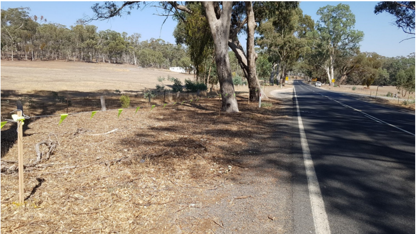
Plate 6. Pyrenees Hwy (Sec 2) Ch 14.720 – 14.880km HHS, Limits of Works, 7 th March 2019.
