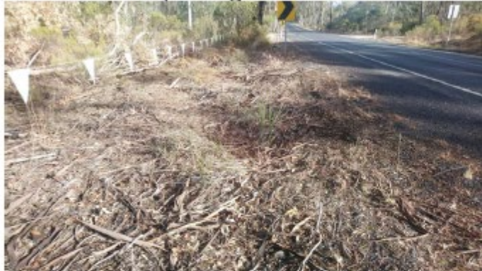
Photo 2: Pyrenees Highway, showing ground cover for fauna habitat (CH 11.115 - CH 11.150 LHS formation widening (fill construction))
