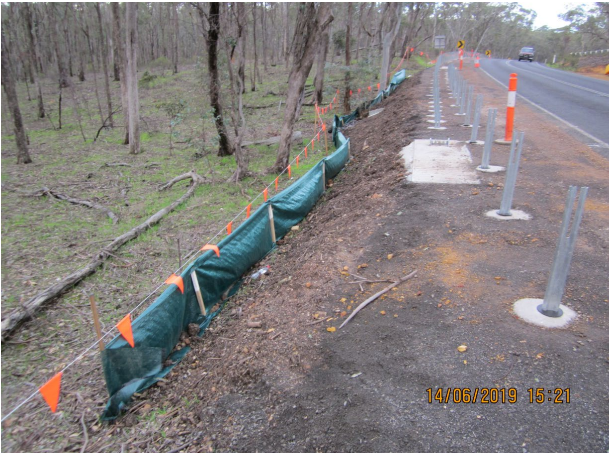
Plate 18. Pyrenees Hwy (Sec 2) Ch 11.880 – 11.405 km RHS, Limits of Works, 14 th June 2019.
