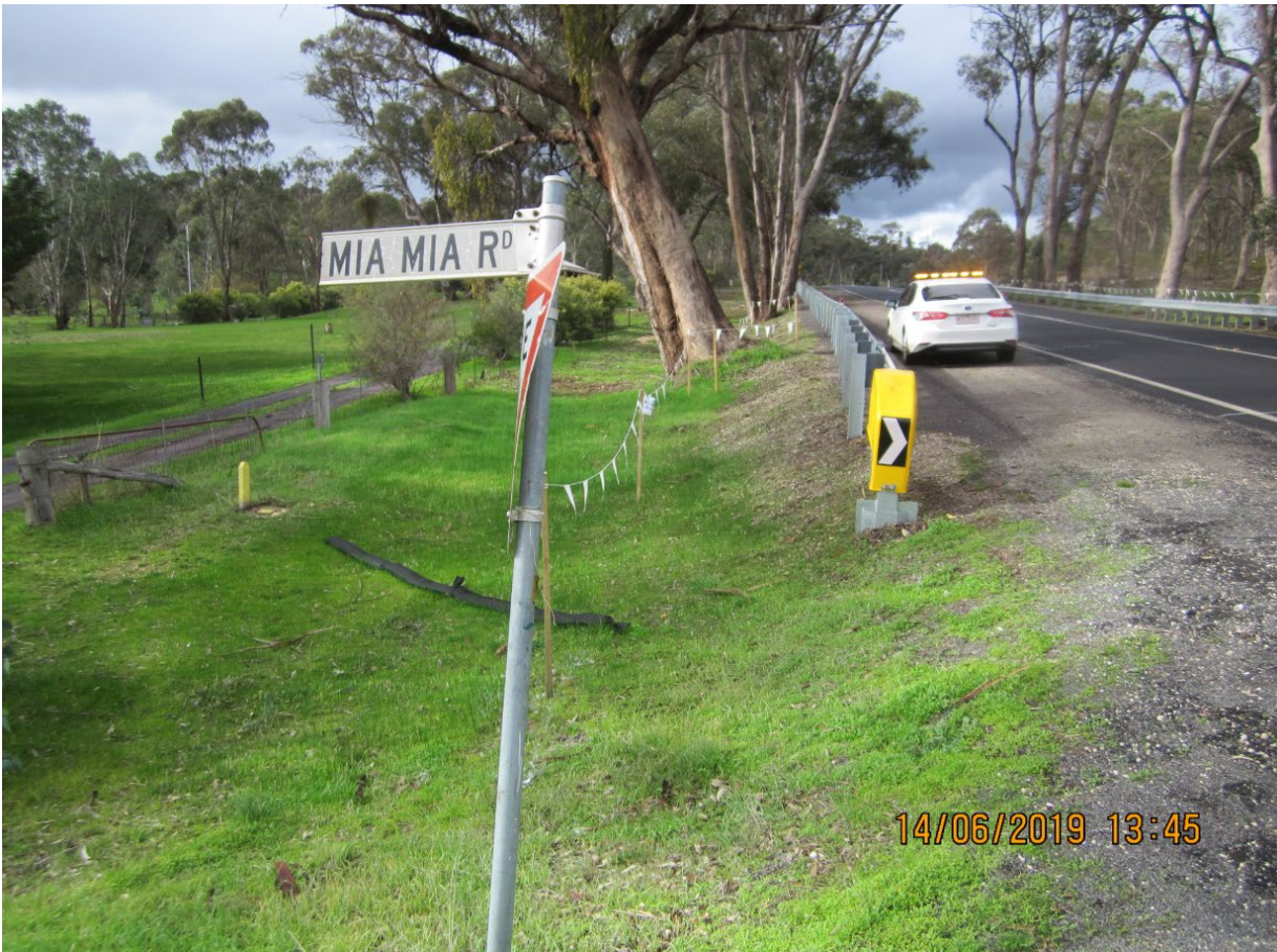
Plate 13. Pyrenees Hwy (Sec 2) Ch 14.800 – 14.705 km RHS, Limits of Works, 14 th June 2019.
