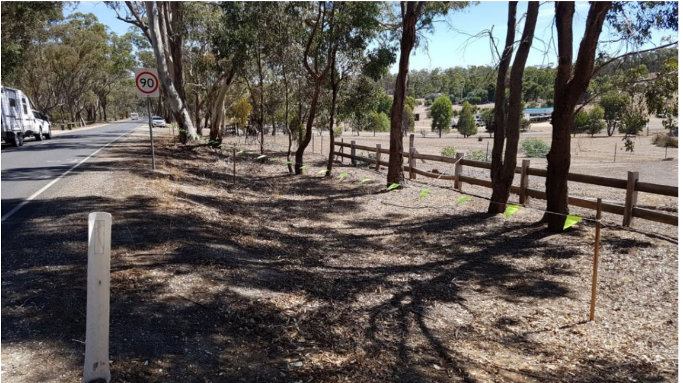
Plate 5. Pyrenees Hwy (Sec 2) Ch 14.000 – 14.070km RHS, Limits of Works, 7 th March 2019.
