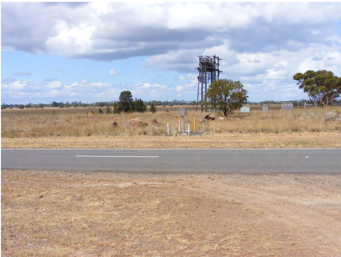
Gantry over railway at Bulban Rd
