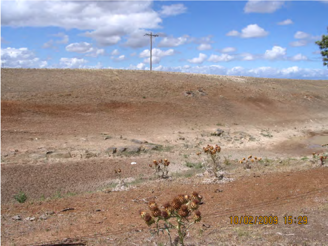
Dam at Ballan Rd
