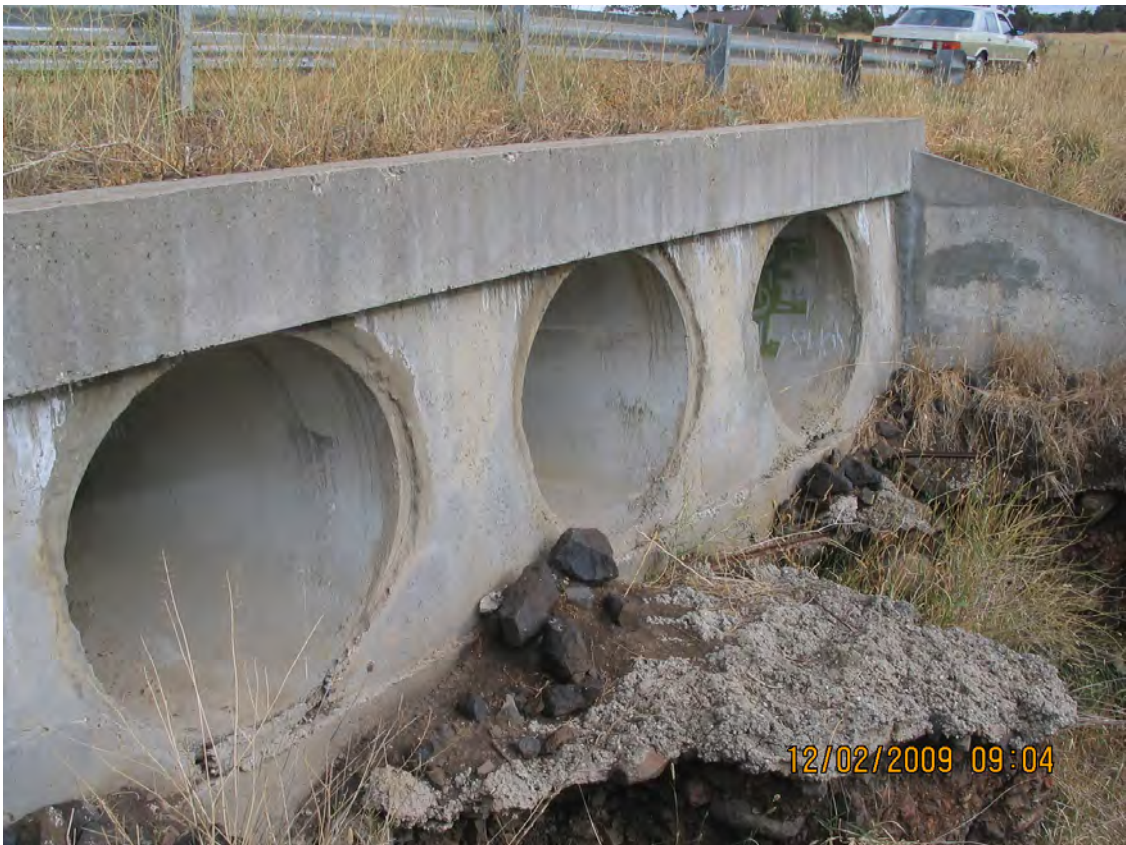
Culvert on Morefield Ct
