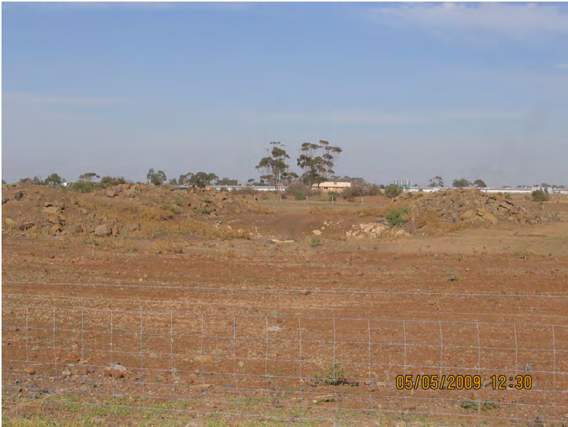
Dam on Middle Road – showing non-rippable basalt in dam bank
