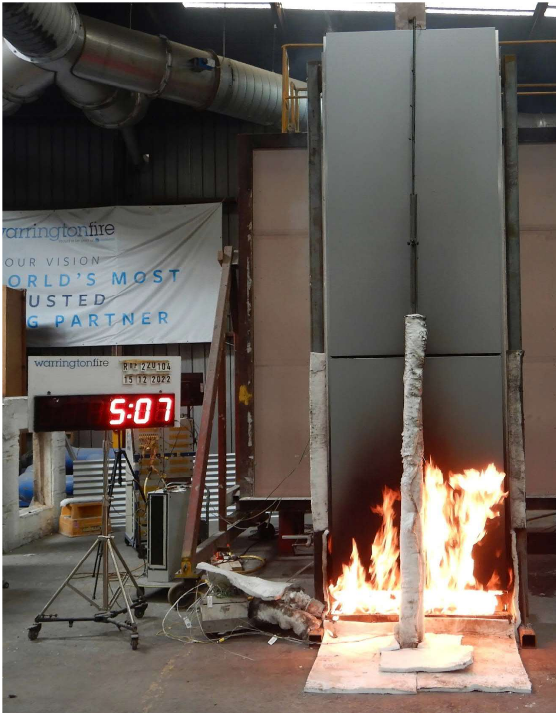
Figure 10 The specimen 5 minutes 7 seconds into the test (burner output at 100 kW)
