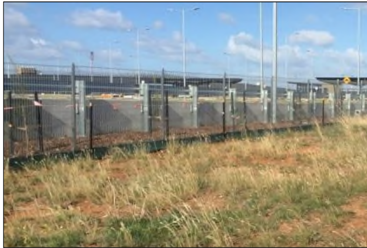
Plate 3. New permanent wire fence delineating the railway station site and the offset site (Ecology and Heritage Partners 23/05/2016)
