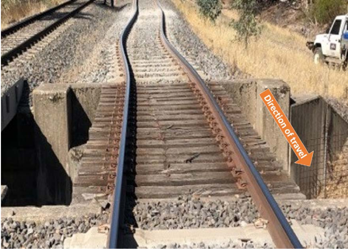
Figure 3: Track misalignment photographed at 1710 on 21 January, after derailment.
