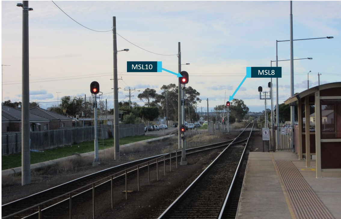
The picture shows signal MSL10 adjacent to the Geelong-end of Marshall Railway Station. Signal MSL8 is identified in the distance, closer to the Marshalltown Road level crossing. Source: Chief Investigator, Transport Safety (Vic)
