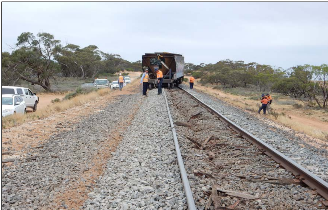
Figure 3: The derailed trailing wagon and track damage
