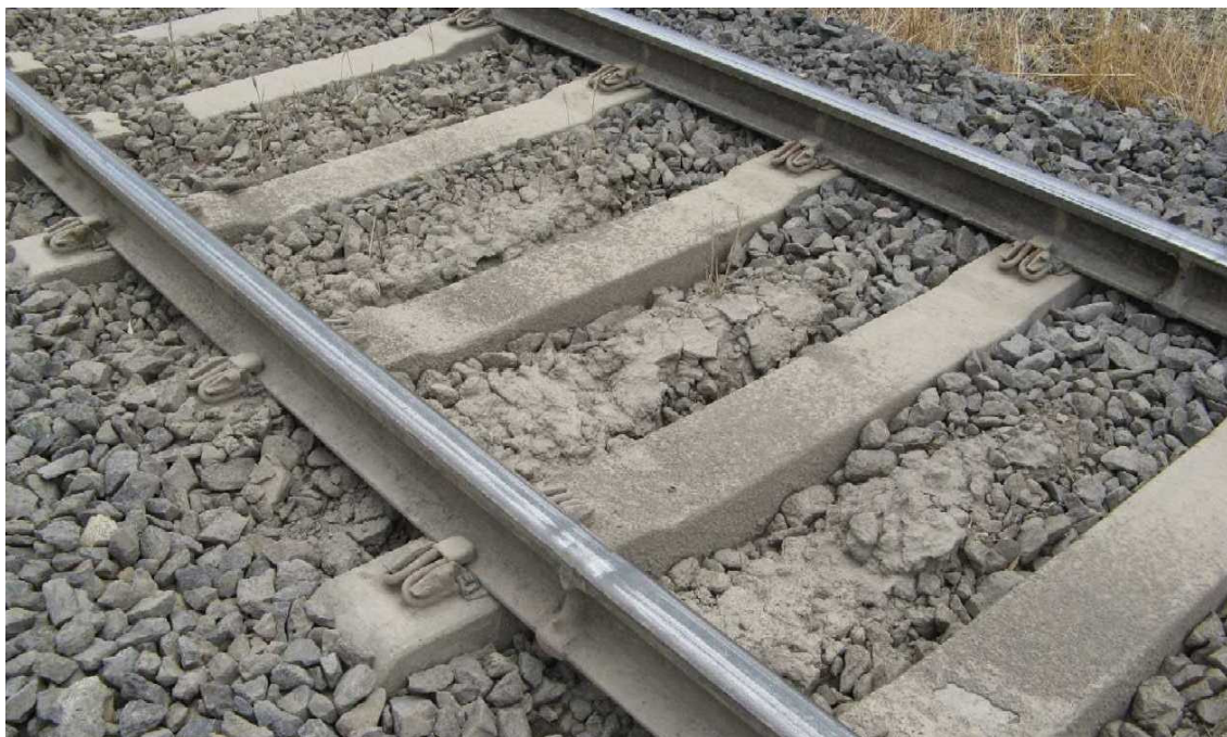
Figure 9 – Repaired track 10-15 metres south of the level crossing (photograph November 2009)
