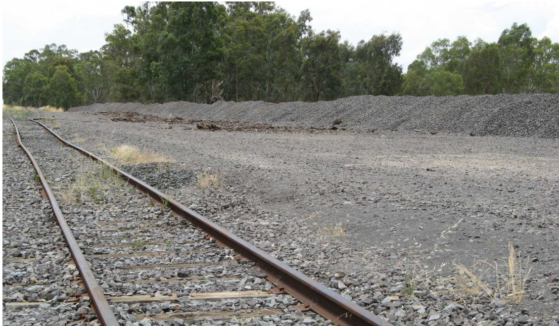
Figure 3 – Violet Town siding, showing ballast stockpile
