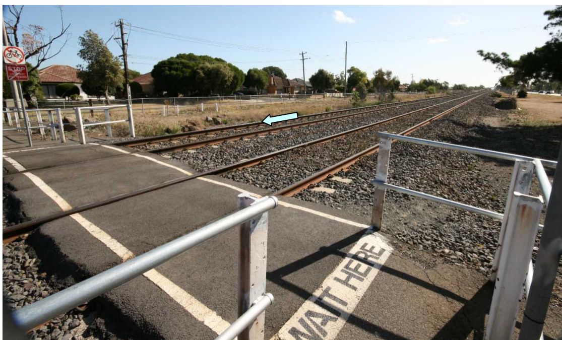
Figure 1. Pedestrian crossing viewed from direction of pedestrian approach
