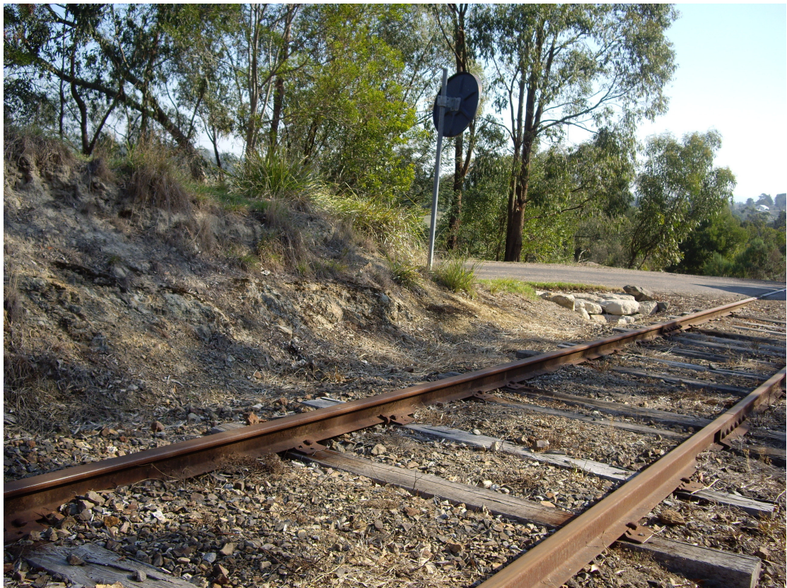
Figure 2 - Rail approach view of level crossing
